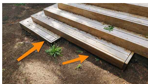
Would to soil contact
