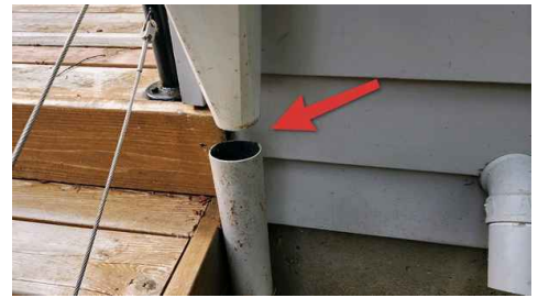
Extend downspout into rain drain
