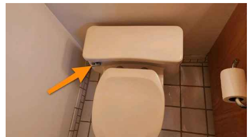
Monitor flashing mechanism
