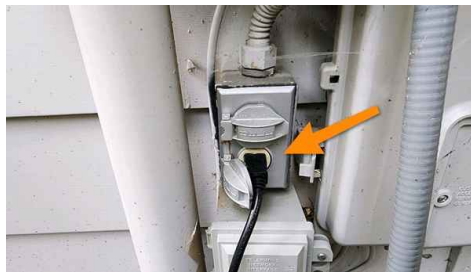
Upgrade outlet box
