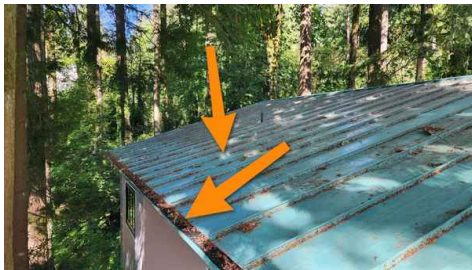
Clean roof and gutters
