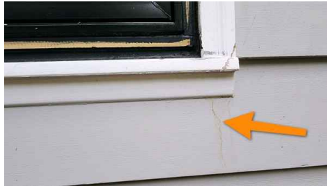
Stains below window
