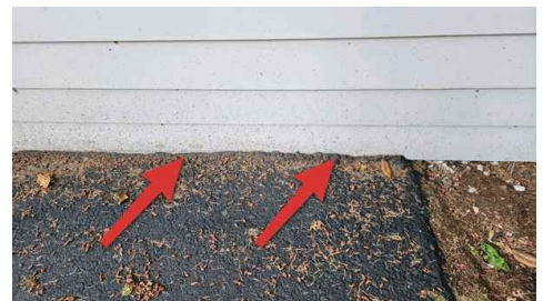
Inadequate clearance
