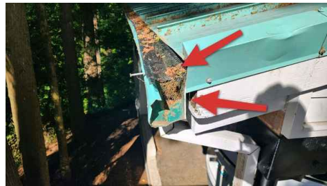
Install cap and clean downspout connection
