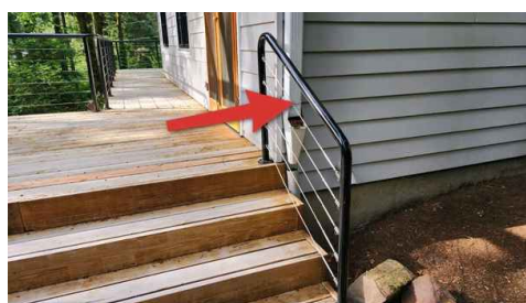
Loose guardrail
