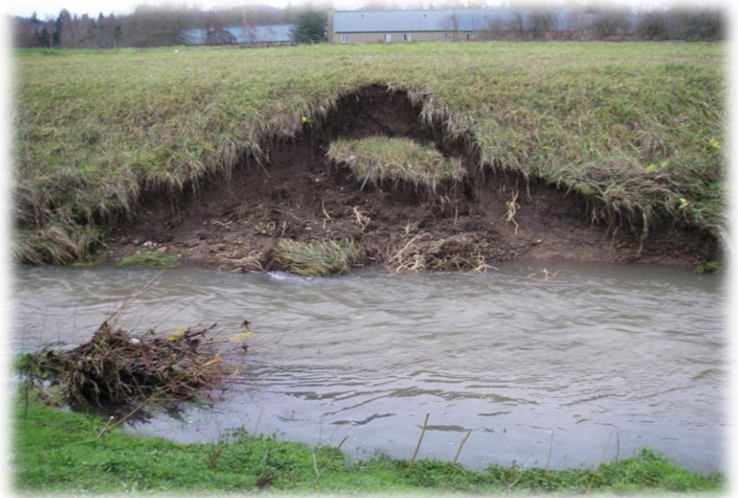
Bank failure along Amazon Creek (2010)
