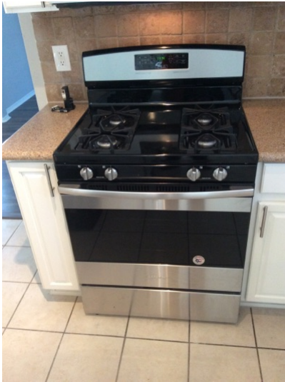
Amana gas range, NO ANTI TIP DEVICE INSTALLED
