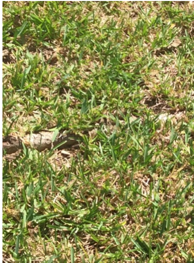
Roots above ground present trip hazards in the front yard
