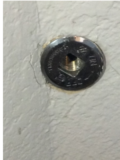
Gas valve for fireplace adjacent to the fireplace. T-wrench was not found
