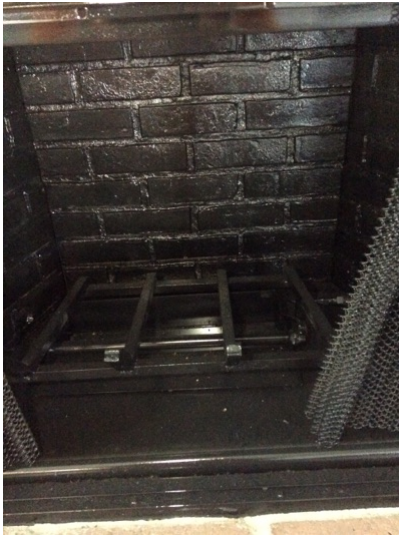
In fireplaces with natural gas, it is required the damper be fixed in a permanent open position. This is done properly on this fireplace
