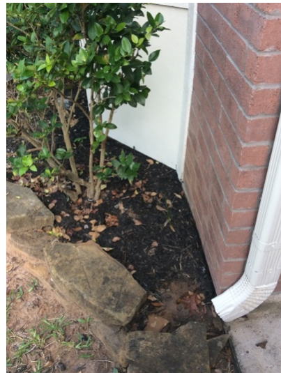
Maintain 6" distance between grade and siding
