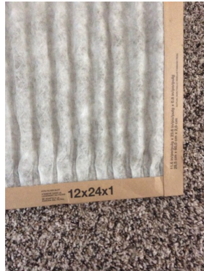
Upstairs return air filter size, 12 x 24 x 1
