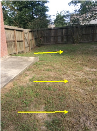
Water properly drains away from the structure
