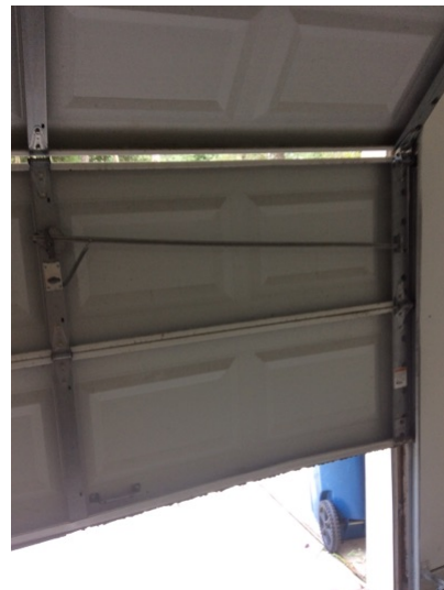
Garage Door Manual Lock must be unlocked and deactivated in the presence of the automatic operator
