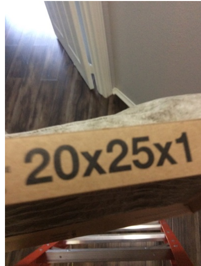
Hall return air filter size, 20 x 25 x 1
