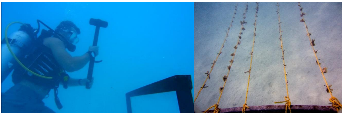
Fig. 16. Steel angle iron “staples” were inserted into the sand in pairs, each separated by 10 m (right) and five nylon ropes were secured between the staples (left).
