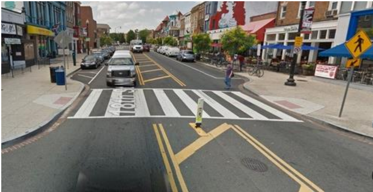
Figure 17: A curb extension and crosswalk at an uncontrolled intersection in the Adams Morgan neighborhood of DC.
