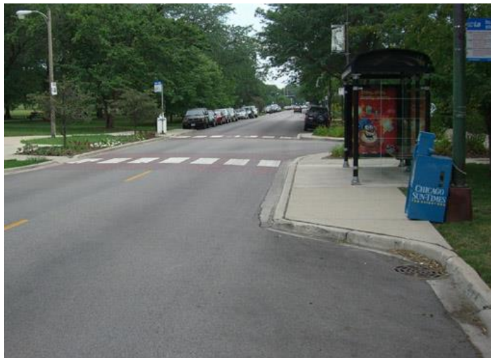
Figure 20: Example of a bus bumpout that allows safe ADA access for riders
