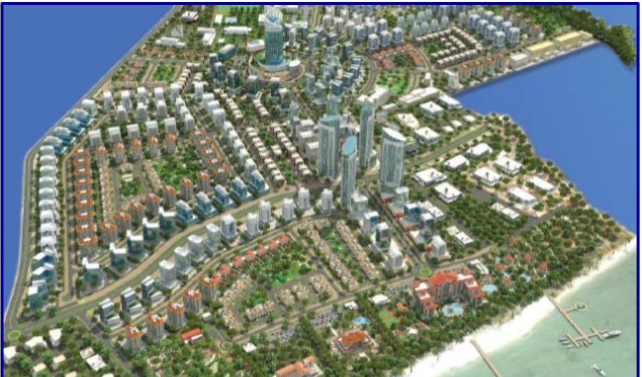
Figure-19: A bird's eye view impression of the proposed Uptown Kawe Satellite City which consists of a 700m stretch of white sand beach linked to the Indian Ocean
