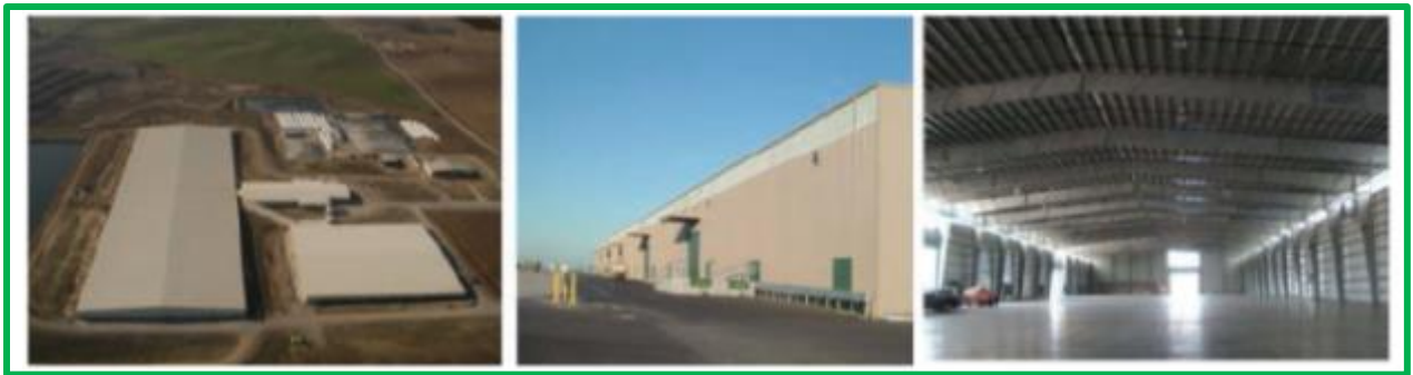
Figure-14: Illustration of Rehabilitated Grain Storage Silos
