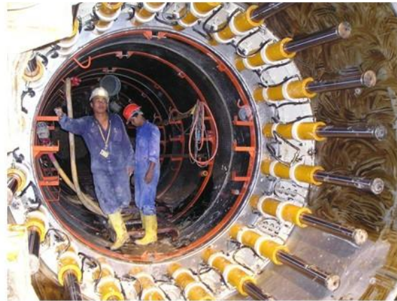
96" RCP PVC lined x 1,000 ton IJS
