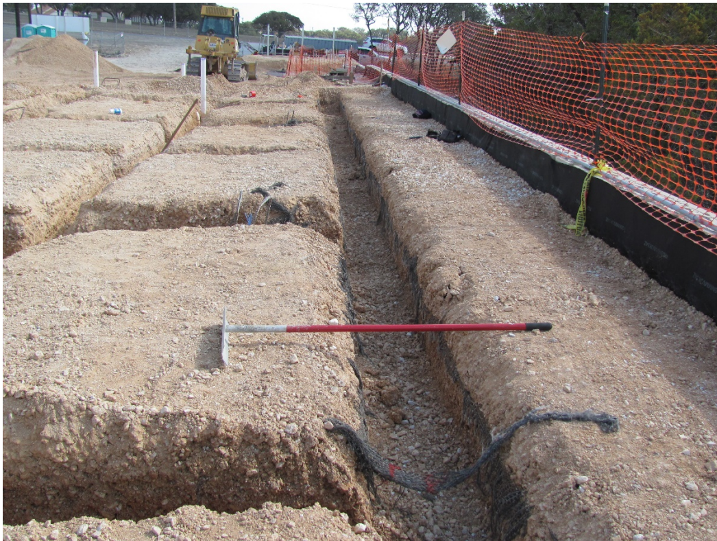
EXHIBIT 8 – APPARATUS BAY – BEAM TRENCHES 01.29.20210
