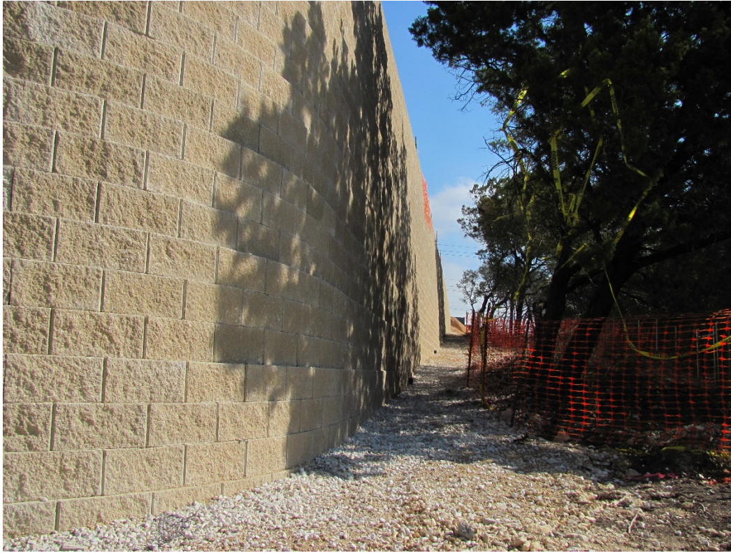
EXHIBIT 5 – RETAINING WALL BLOCK COMPLETE 01.29.2021
