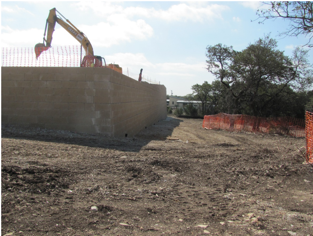
EXHIBIT 4 – RETAINING WALL BLOCK COMPLETE 01.29.2021
