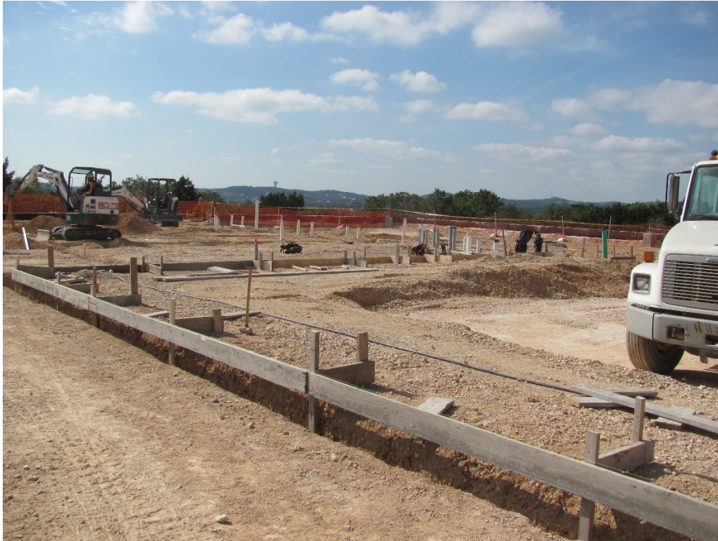
EXHIBIT 7 – MAIN FOUNDATION – CONCRETE FORMS 01.29.2021
