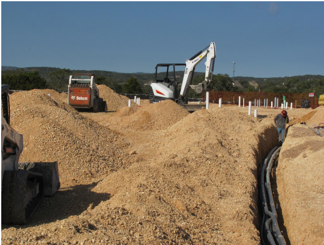
EXHIBIT 2 – DRY UTILITIES – BUILDING TO GENERATOR PAD 01.26.2021
