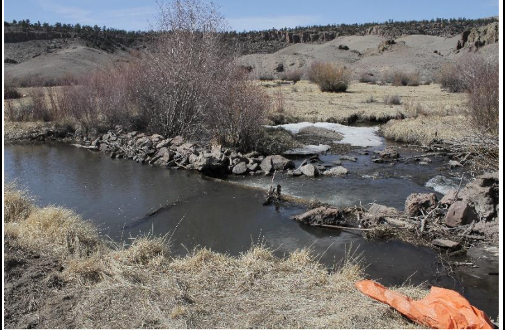
Diversion dam looking downstream
