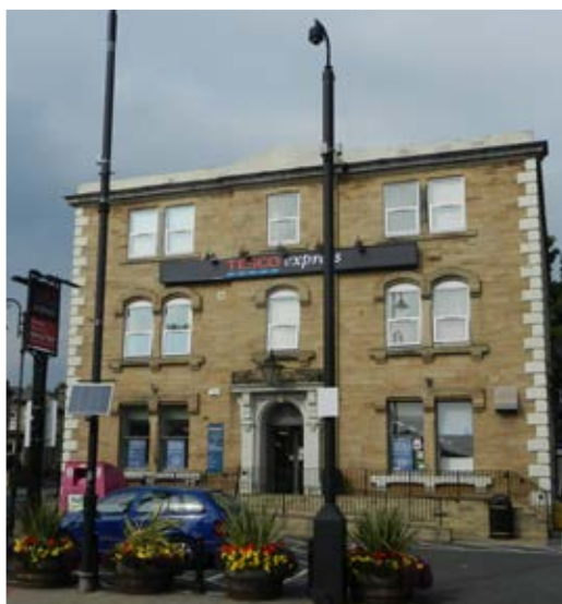
Huddersfield Road shopfront
