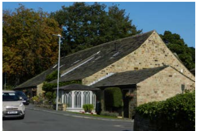
Figure 60: Main barn to Hall Farm
