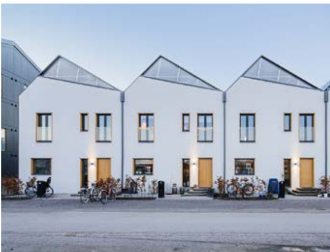
Figure 44: Asymmetrical roofs with photo-voltaics aligned for solar orientation in these 'solar terraces'
