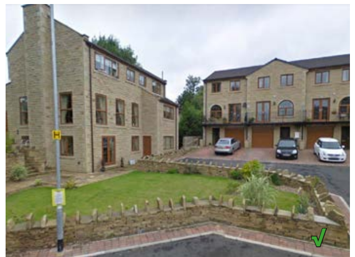
Development at Greenside Close has sympathetic materials, well proportioned windows and is of a comparable scale
