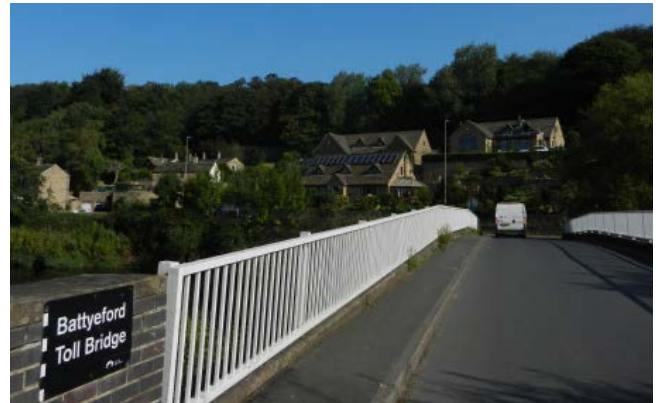
Battyford Toll Bridge (Halfpenny Bridge)
