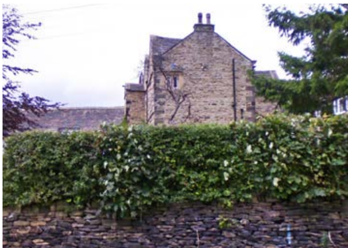
Figure 85: Norththorpe Hall boundary wall
