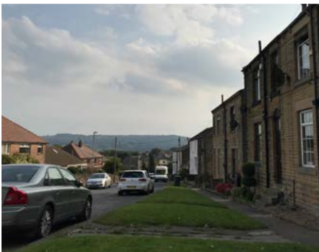
Figure 21: Northorpe Lane lacks boundary walls but has a green verge with footpath beside front doors
