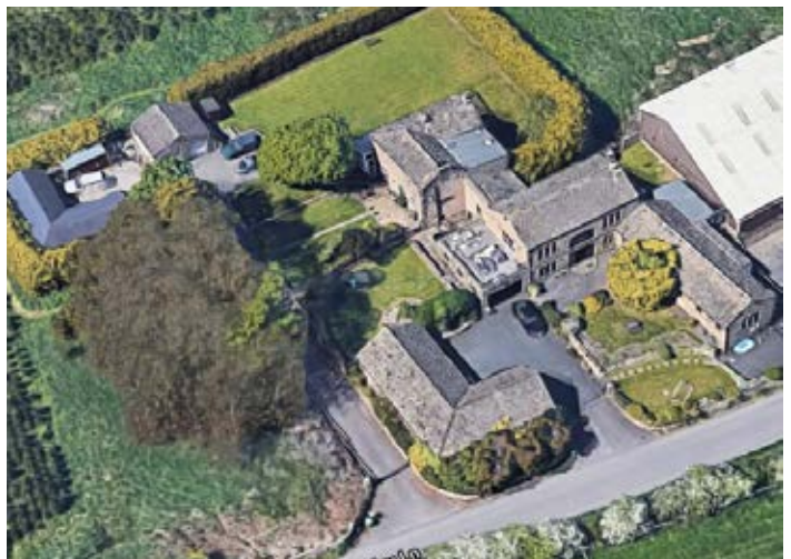
A typical complex of farmhouse and related buildings that form courtyards and sit within a variety of planting including a stand of trees which can help to settle visually and reduce exposure to strong winds
