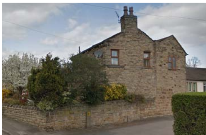
Sandstone terraces / buildings are predominant along Greenside Road, and together with the stone walls
