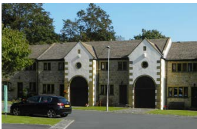
Figure 42: New houses on Towngate (Mirfield) and Covey Clough Court (Upper Hopton) introduce a varied but attractive and complementary palette of materials and detailing. In the former case this is strictly contemporary, whereas around the conservation area motifs and detailing may
