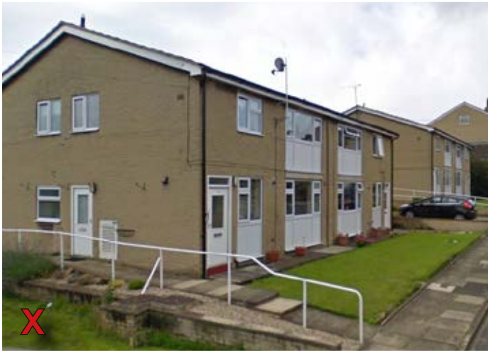
Later homes in Lower Hopton of a different scale, with different proportion windows and openings to the traditional terraces
