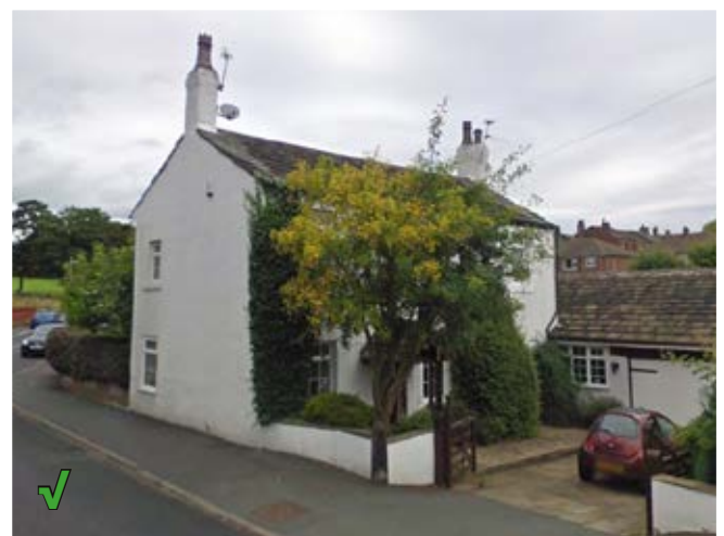
Figure 34: Cottage set at right-angles to the street with wall, gate, courtyard planting and retained tree
