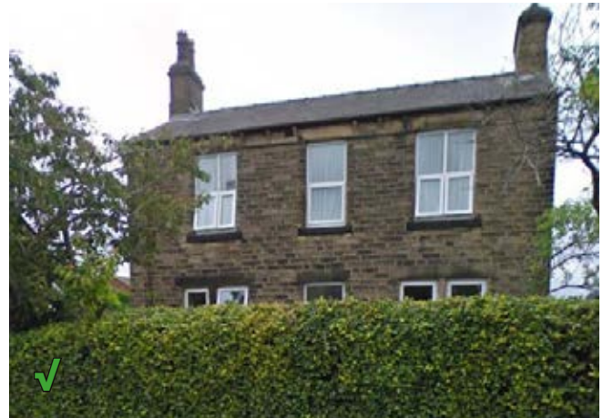
Figure 33: Hedgerows provide privacy to this cottage
