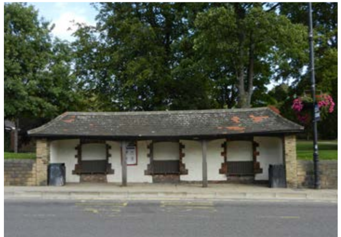
This well built and solid bus stop is pleasantly fitting with the town centre aesthetic
