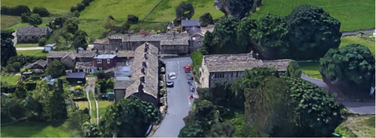
Figure 102: Northgate/ Hollin Hall hamlet is a cluster of dwellings that forms a key gateway
