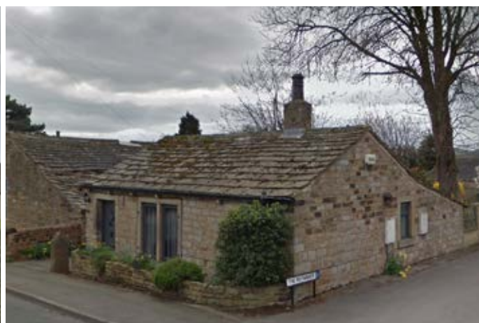
Single storey stone cottage conversion at junction with the Reynards
