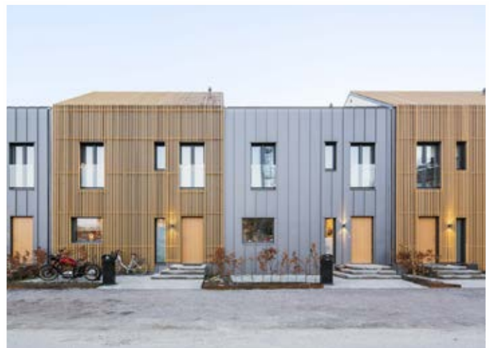
Figure 45: Cladding and roof angle varied to provide visual interest and aligned to north - south orientation
