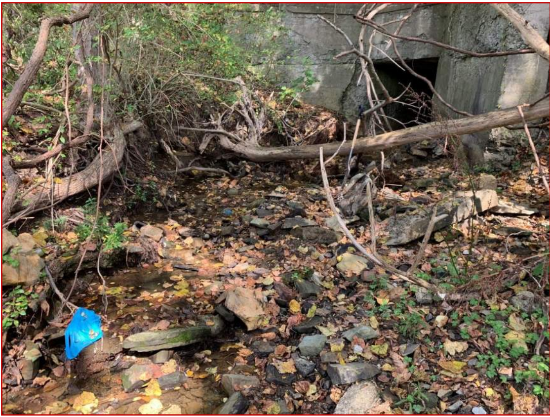
Photo 1: UNT 1 to Jacks Run – Facing Upstream (9.17.19)
