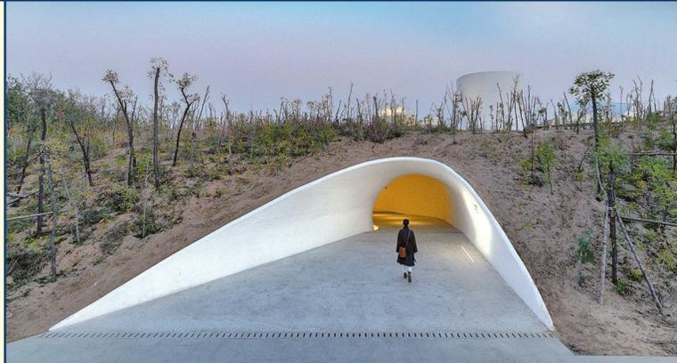
The existing dune was excavated and the structure was erected with steel columns encased in concrete, with steel micro-piles transferring the vertical load to bedrock beneath the brick walls. The atrium walls are 18 in. thick. To prevent condensation, engineers devised thermally broken connections between the new steel elements and the existing masonry walls. The sand-covered roof helps to keep the interior cool in the summer.
