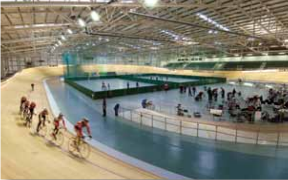
Reznor Low Intensity, Tubular, Radiant Heater in a Sports Complex
