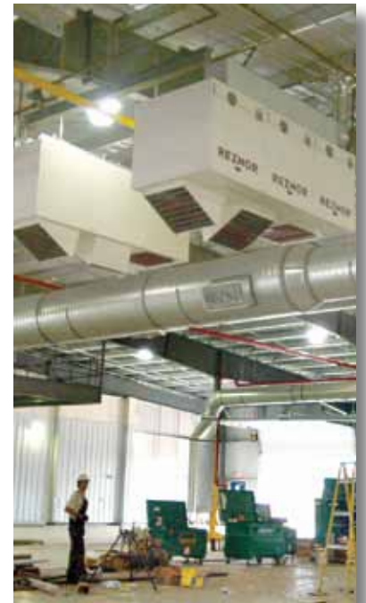
Model LDAP Gas Fired, Air Turnover Heater
