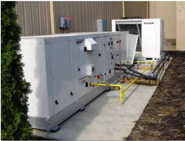
Split System consisting of a Model RDH Air Handler and Model MASA Condensing Unit
