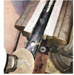
**2)** Locate the rivet end and grind it down to expose the rivet shaft.
