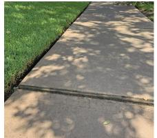
As our community ages, more sidewalk repairs will be required. The primary culprit that causes sidewalks to fail is tree roots. Trees will get water wherever they find it; if that is under your sidewalk, that is where they go. The result is one or more concrete panels sinking, resulting in uneven sidewalks. Perhaps water "puddles" on you walk like this. This could indicate that section has sunken and needs to be raised before it becomes like the one above.
