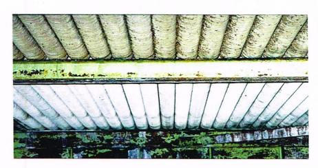
The Foaminator System consists of specialized chemicals and equipment. The Foaminator pumping system is used to form and inject a dense heavy "shaving cream like" foam into and around the fin fan coils. The chemical foam dissipates slowly while removing the deposits from the fin surface. The Foaminator will remove severe accumulations of hard mineral deposits such as calcium, as well as dust, dirt, and other deposits.
