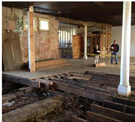
Phase One work included structural repair of the wood floor framing.
