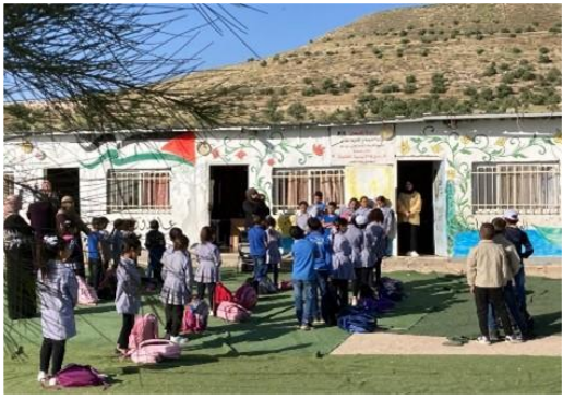
Photo: Jubbet ad-Dhib school before it was demolished
