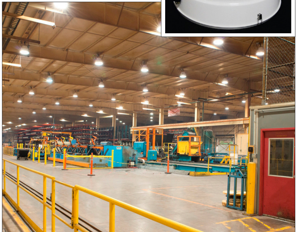
ArcelorMittal Marion. We replaced 1000W High Bay Lights with 630W and 315W Best Lights Fixtures. $88K Per Year in Electrical Savings – More Light – Two Thirds Less Maintenance.
