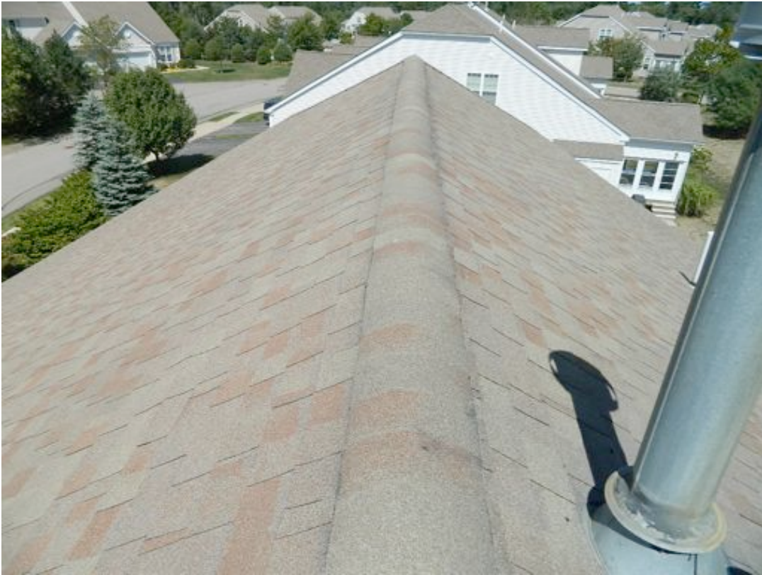
TYPICAL SHINGLED-OVER RIDGE VENT
