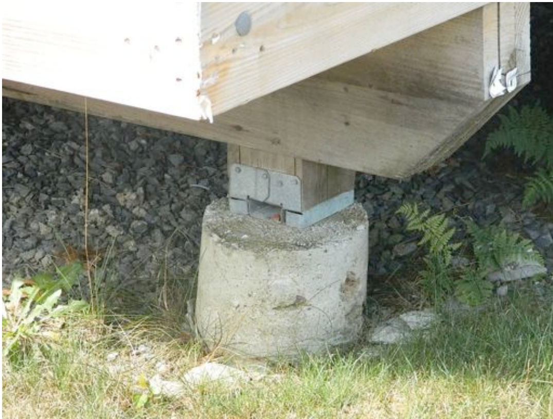
THE DECKS REST ON POURED CONCRETE FOOTINGS
