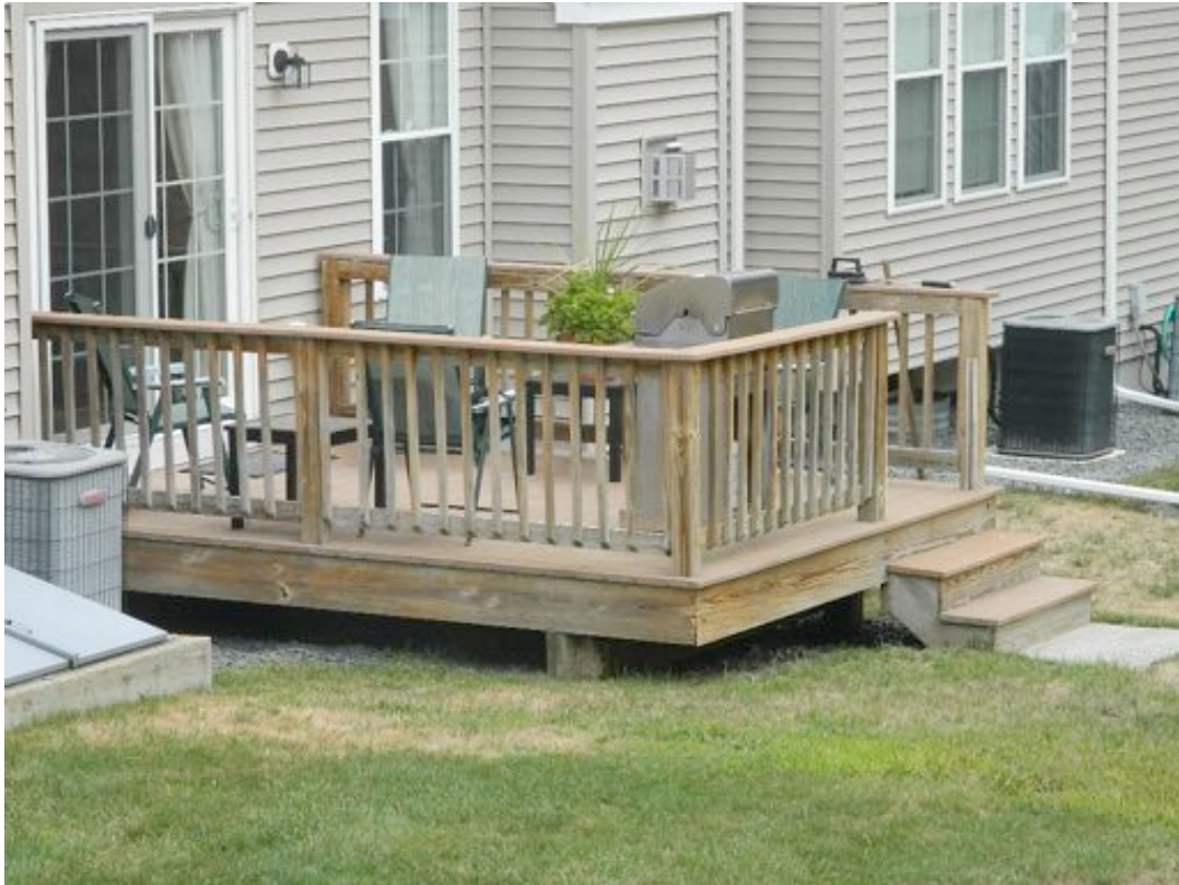
TYPICAL GRADE-LEVEL OPEN WOOD DECK
