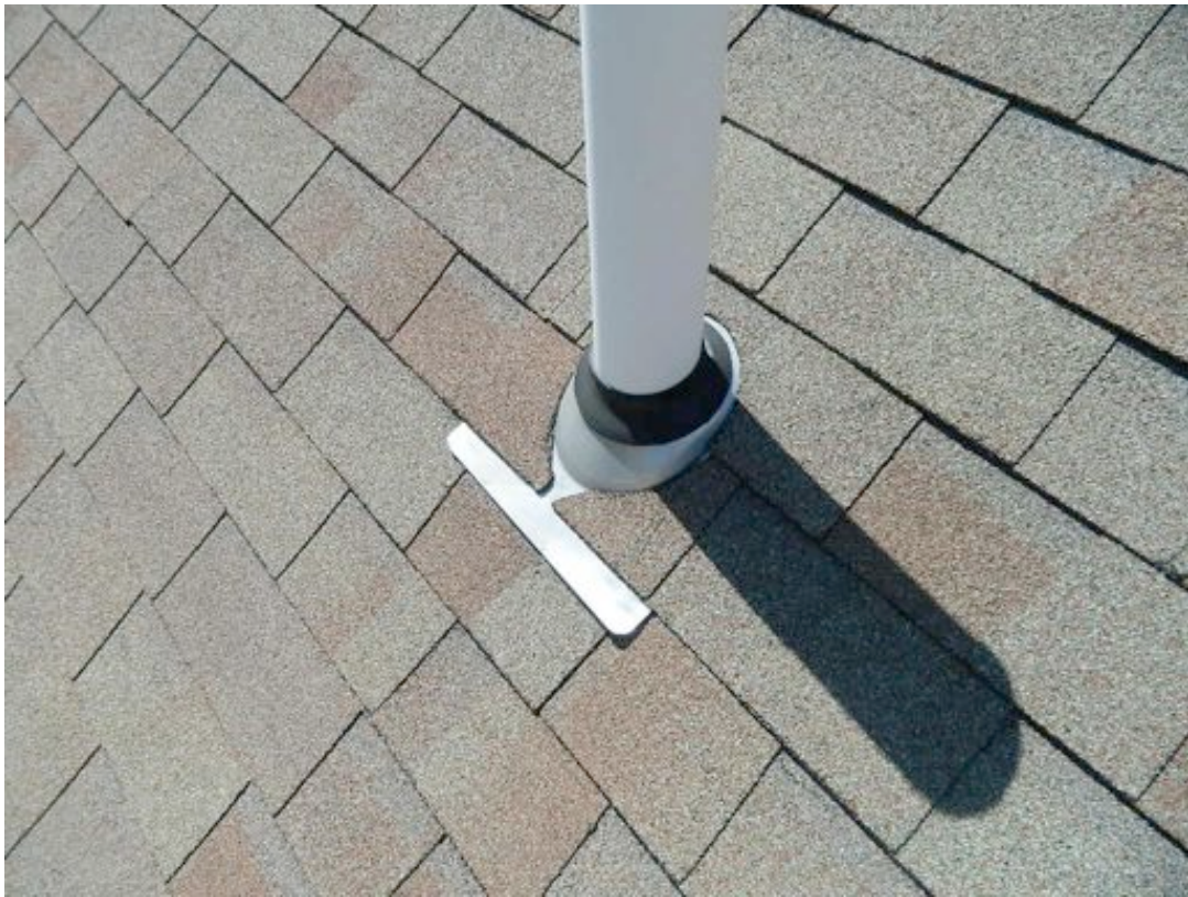
TYPICAL NEOPRENE/ALUMINUM PIPE FLASHING
