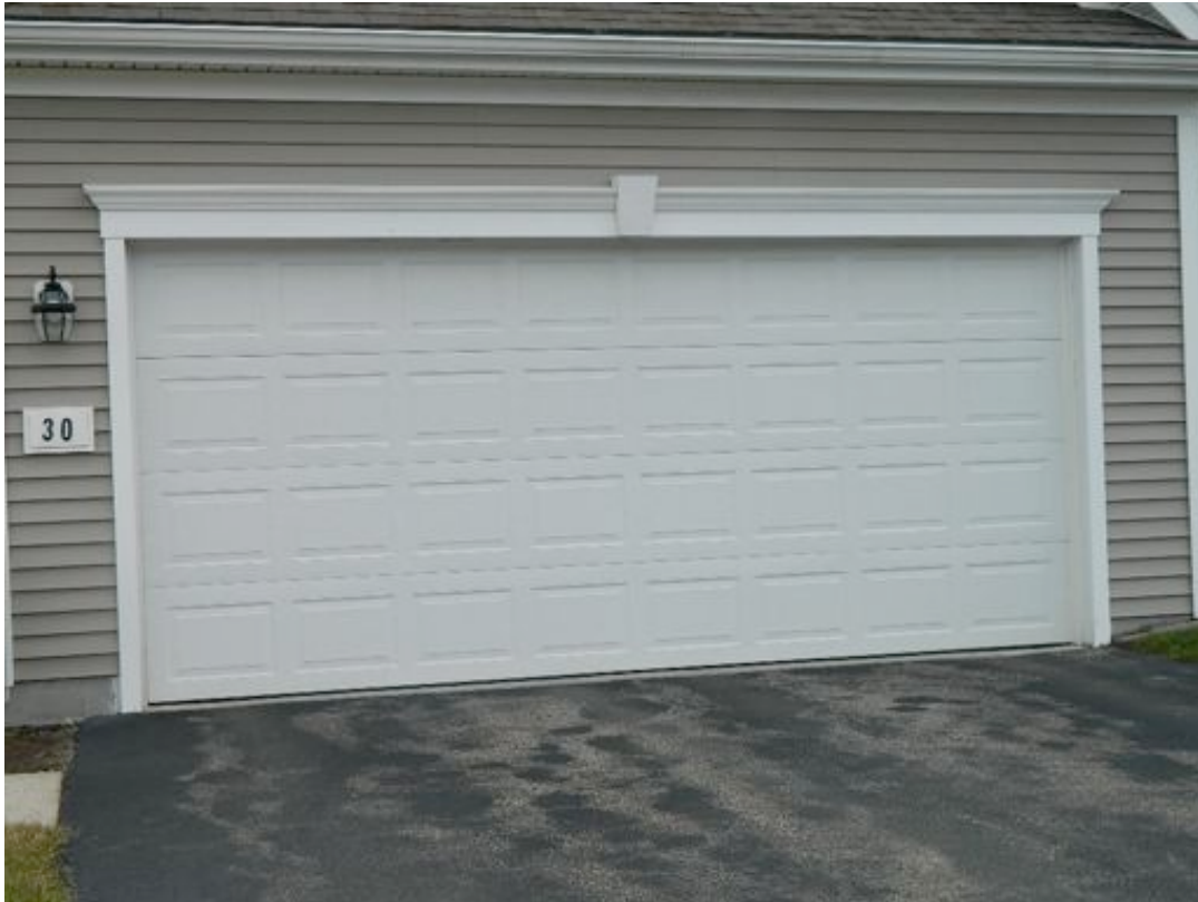
TYPICAL 16 X 7 INSULATED METAL OVERHEAD DOOR
