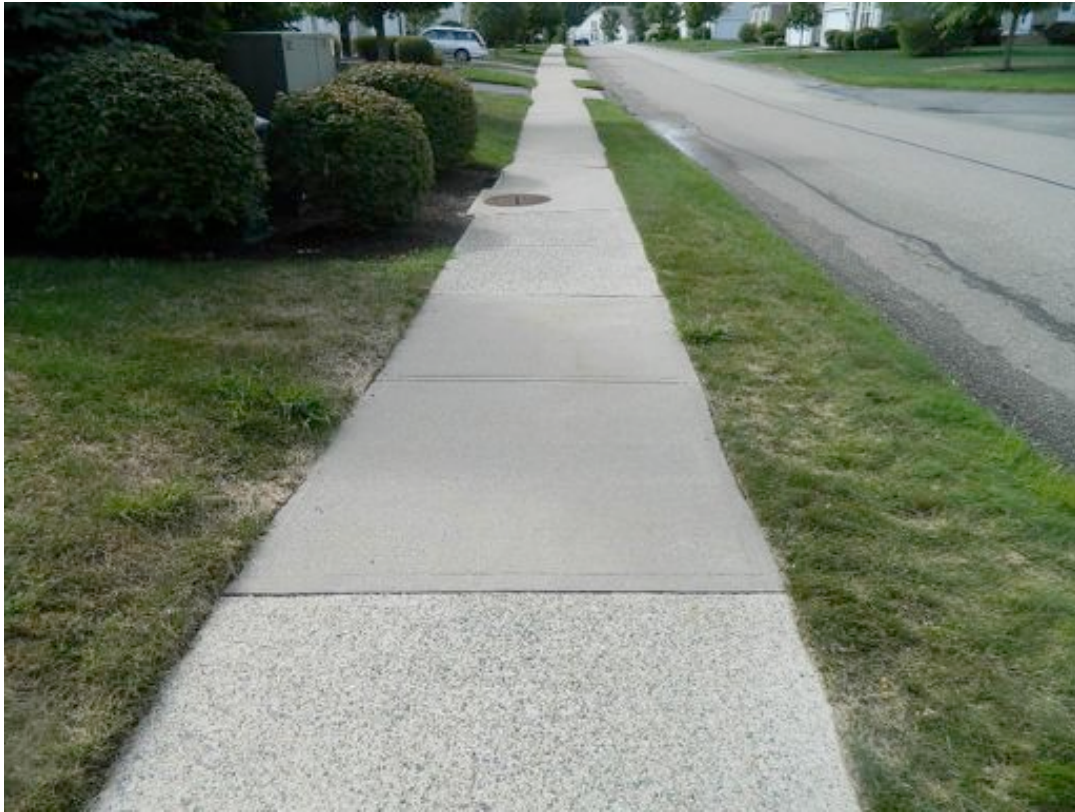
SOME INDIVIDUAL PANELS HAVE BEEN REPLACED
