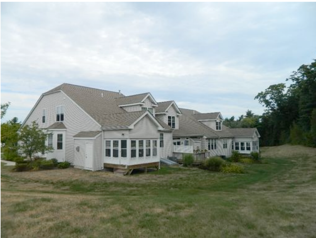
REAR OVERVIEW OF A TYPICAL BUILDING AT SPYGLASS LANDING
