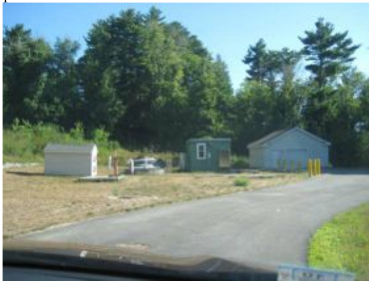
Wastewater Treatment Building & under ground Tanks
