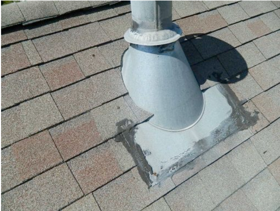
TYPICAL TYPE B GAS VENT STACK FLASHING
