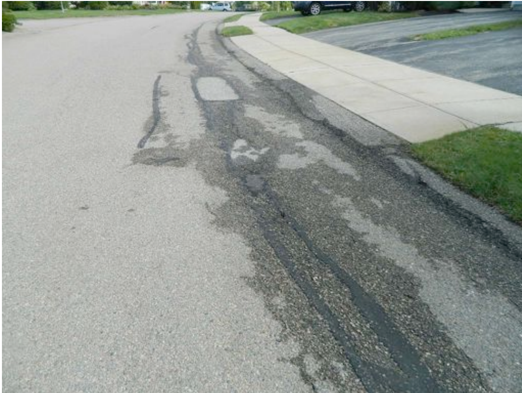
DRIVEWAYS ON THE SIDEWALK SIDE HAVE CONCRETE WALKS
