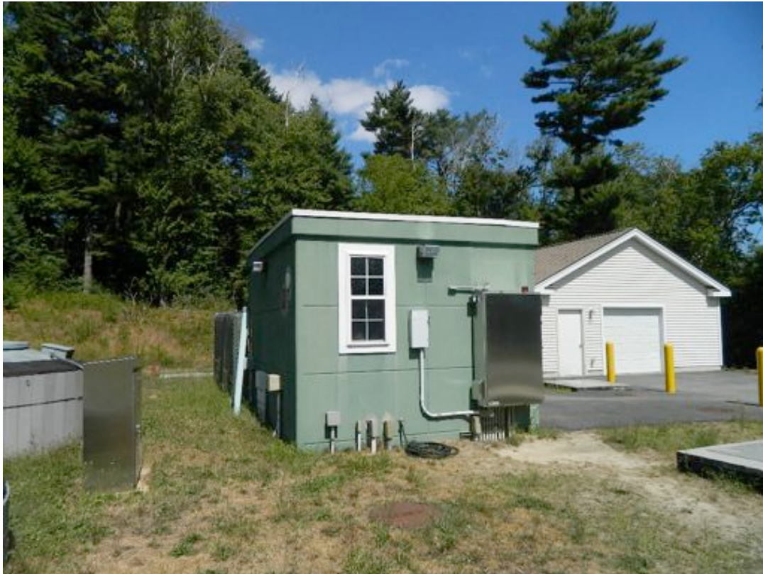
WWTP CONTROL BUILDING
