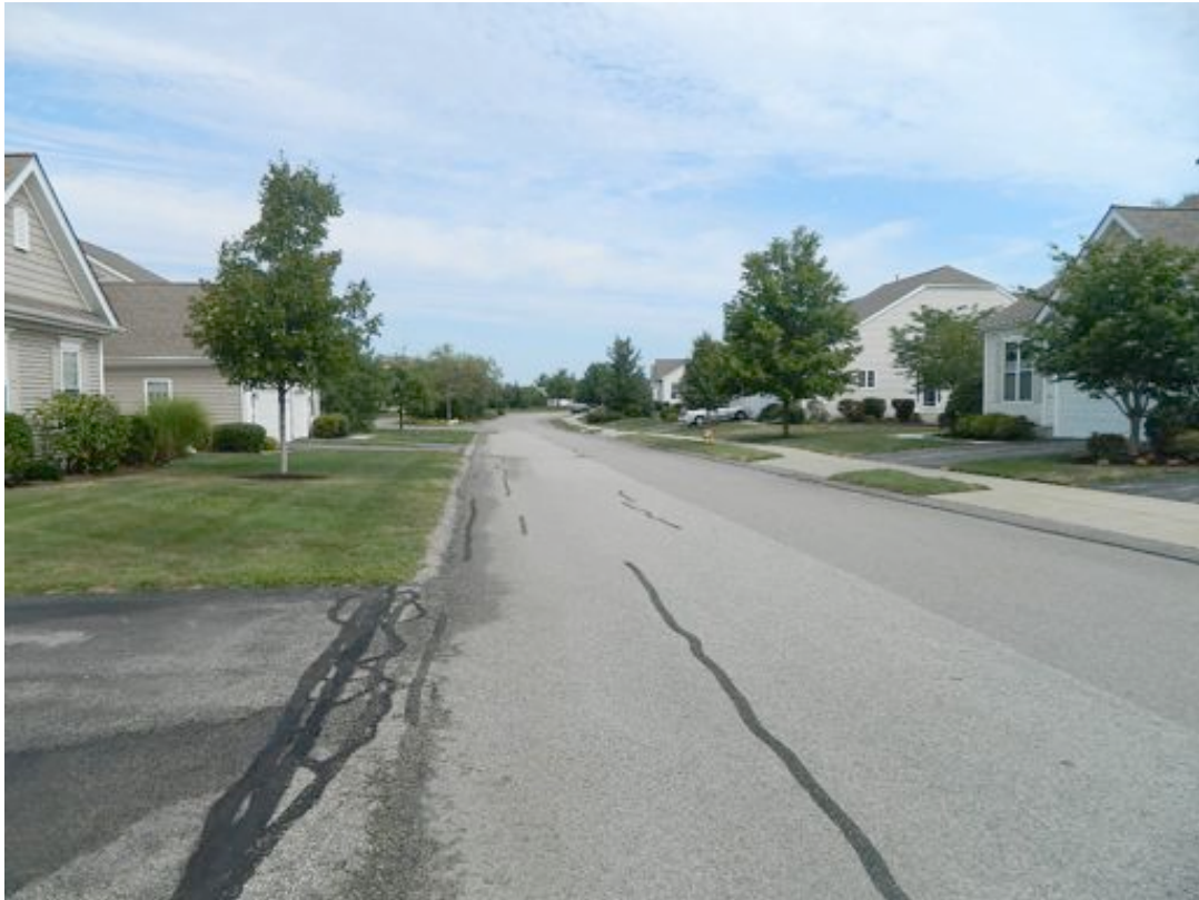
THE ASPHALT PAVEMENT IS IN "AGE APPROPRIATE" CONDITION
