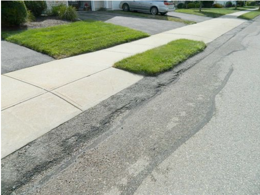
MOST OF THE CONCRETE SURFACES ARE IN GOOD CONDITION
