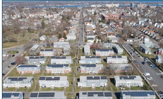
On-Site Rooftop Solar PV
