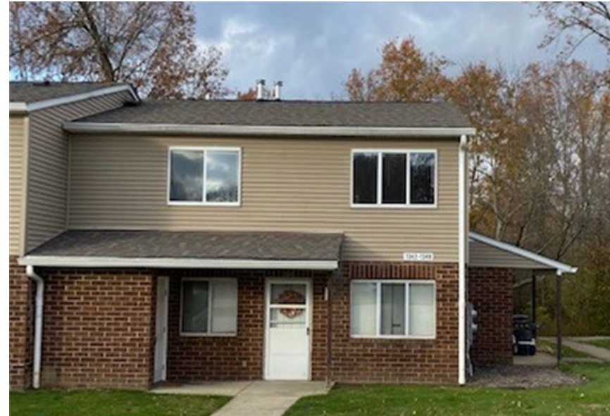
New windows and doors installed in 2021 in Akron, OH
