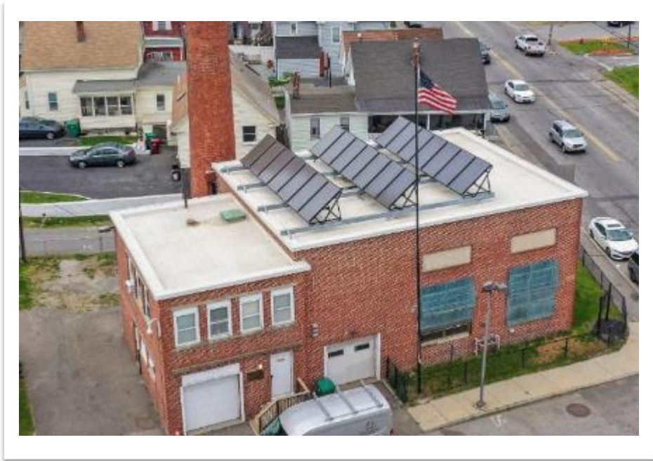
New roofs (here with solar thermal) installed in 2021 in Lowell, MA
