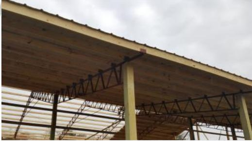
With trusses spaced at apart 10' apart as a standard. you will reduce the number of trusses, materials and labor cost with our quality steel truss system.
