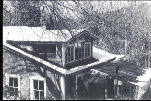
Dormer added 1948 Facing east Mother's room.
