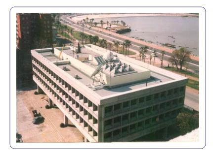
The U.S. Embassy for Uruguay is located in the capital city of Montevideo. The main building is called the Office Building Chancery which is a 3-story concrete framed structure that was designed by I.M. Pei and constructed in the early 1970s. One of the projects that was assigned to PCI under an IDQ contract was the design for roof replacement of the subject building. PCI services also included technical consultation and quality assurance inspections during the roof replacement.
