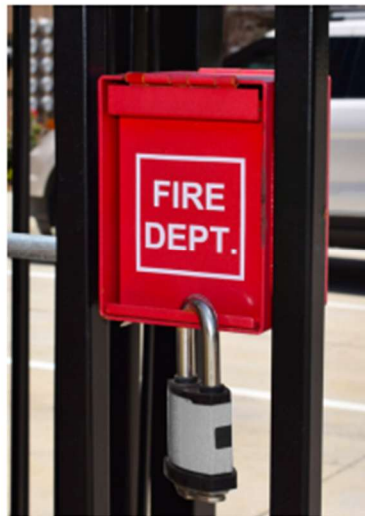
Fire Dept. Access box with Knox® Padlock on front
