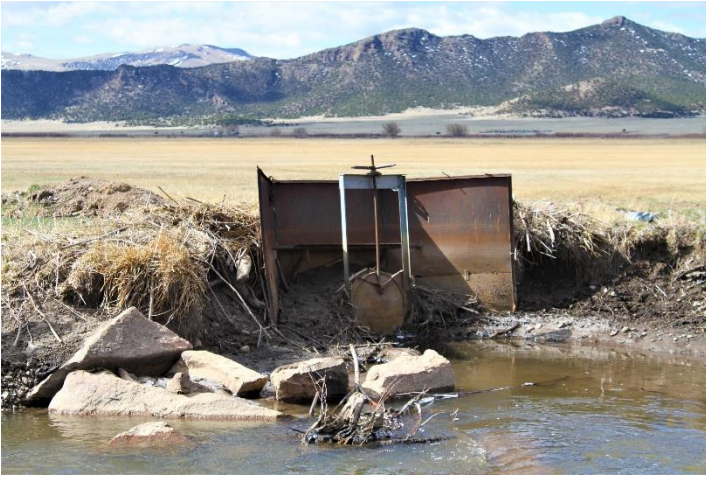
Headgate looking downstream
