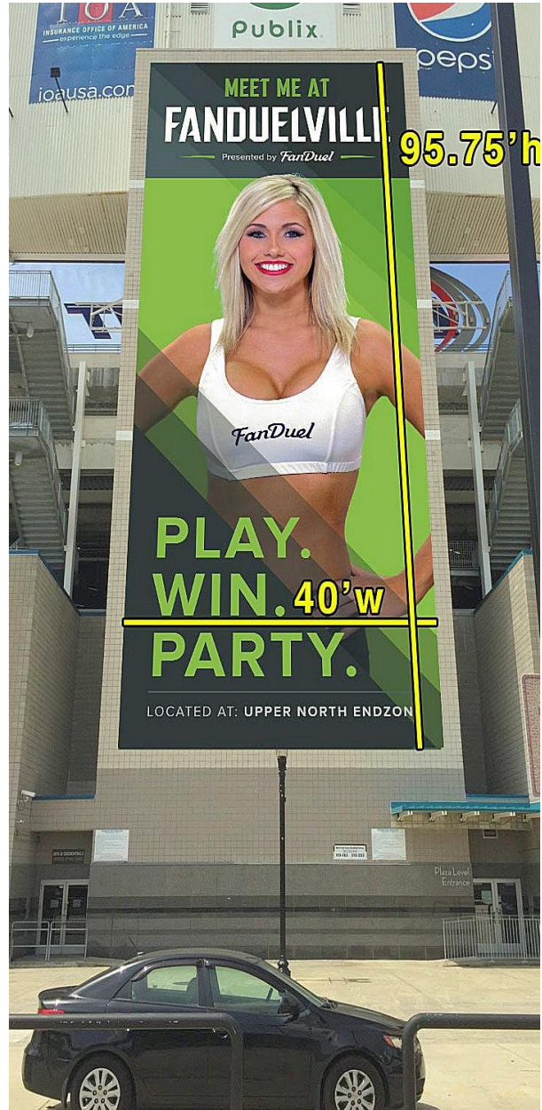
Jacksonville Jaguars 95.75'H x 40'W frame with printed vinyl, installed on the outside wall of the stadium.
