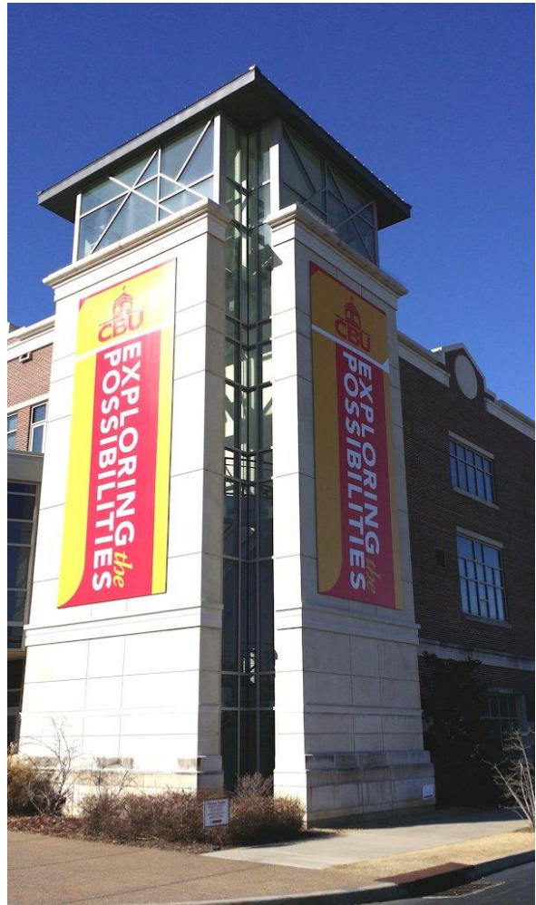
CBU Tower – Two 32'H X 11'W TS44 Frames
