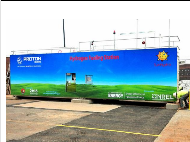
Vinyl banner installed on a 40'W x 9.5'H rigid frame (See on the right) with two windows. This project is the façade on a hydrogen pump.
