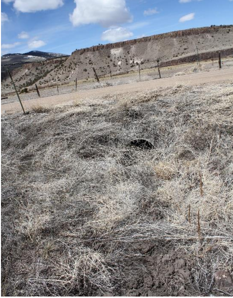
Ditch entrance looking downstream
