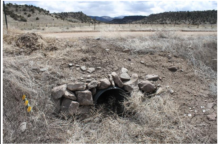
Ditch culvert outlet
