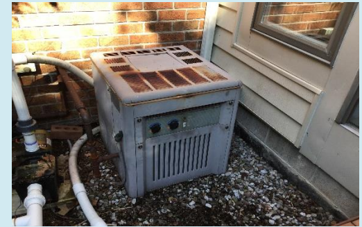
Heater not responding to thermostatic controls at time of inspection. Appears past its serviceable life. Manufacturer date 1994.
