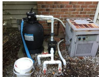
All PVC. No issues noted No Issues noted
