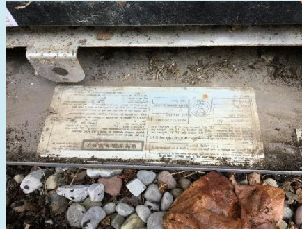
Heater not responding to thermostatic controls at time of inspection. Appears past its serviceable life. Manufacturer date 1994.
