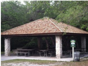
GREYNOLDS PARK RE_ROOF Miami-Dade County Parks & Rec Contract # 96732
