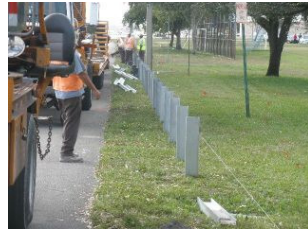
FLATWORK & GAUARDRAIL Broward College Campus Contract #201100001672 #
