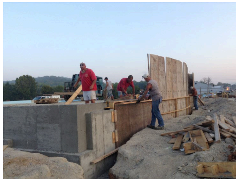
Our "crew" on the bank site beginning another day
