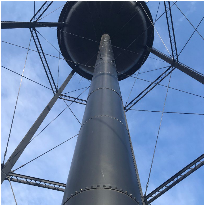
Fair to good condition with minor fading and chalking. Black color/coating holding up fair.
