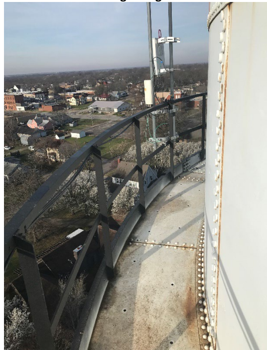
Sidewall and catwalk fair condition with normal chalking, fading and degrading.
