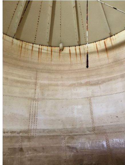
Fair condition with some staining and minor coating failure in the liquid zone. Vapor zone more corrosive and more difficult to blast/coat is why you generally see more
