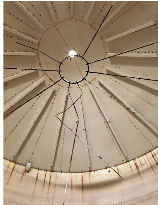
Fair condition with some staining and minor coating failure in the liquid zone. Vapor zone more corrosive and more difficult to blast/coat is why you generally see more
