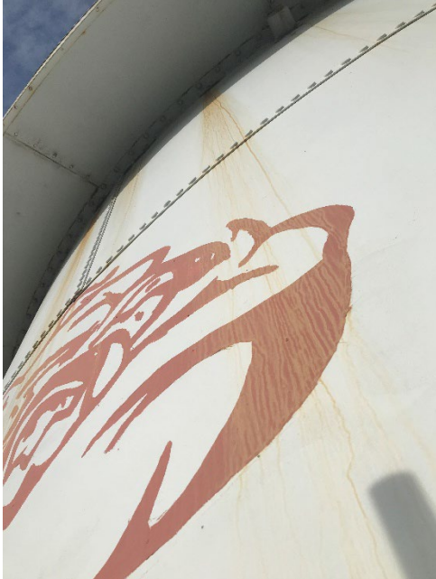
Fair condition with fading, chalking and some staining from the roof eave.
