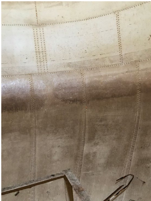
Fair condition with some staining and minor coating failure at bottom of wet riser.
