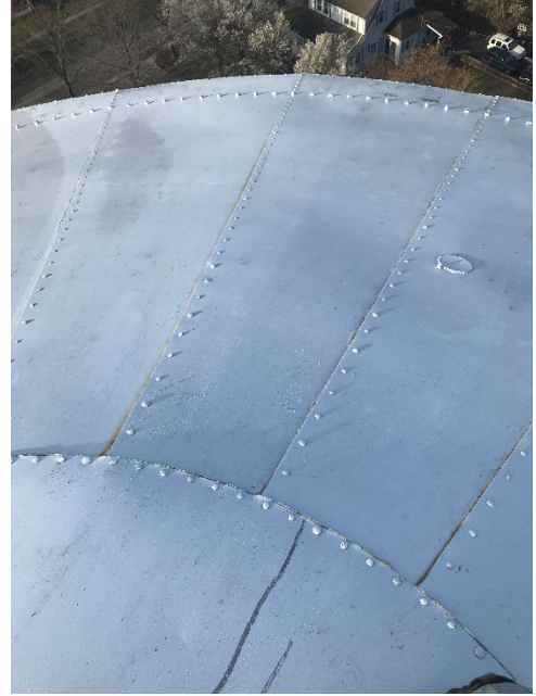
Roof in fair condition with fading, chalking and normal degrading.
