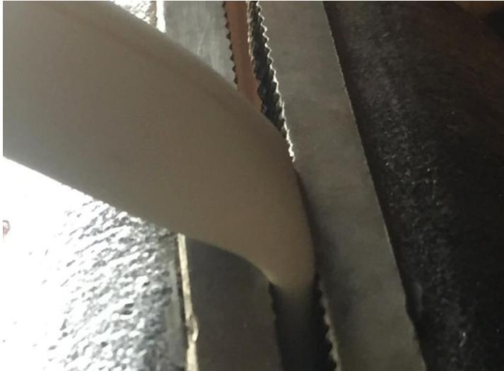
Once the pipe is heated, place the heated end in the vise and quickly squeeze it flat. Don't squeeze beyond just causing the two sides to meet. If you overtighten, you can flatten it out so thin it has no strength, and widens way out beyond what is usable. (Even done properly, the flattened sides may need to be ground back to the diameter of the conduit.)
