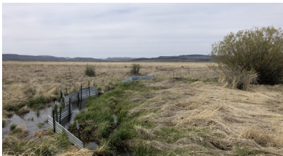
Structure to discourage fish from down-migrating into N. Fork Mahogany Creek 2020.
