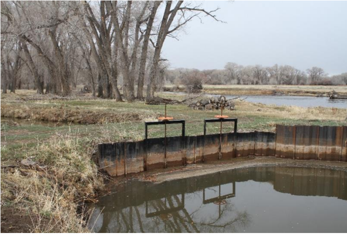
Headgate looking downstream
