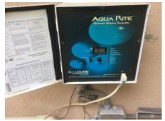
• There is an error message on the salt chlorination system indicating one or more faulty condition. This includes check salt and inspect cell, which may indicate a lack of recent maintenance. We recommend this condition be corrected by the pool service personnel for water chemistry and proper chlorination
