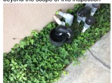
• The drain for the filter backwash is required to have an air-gap of at least two inches above the flood rim of the drain. The discharge pipe enters the drain, and could cause a backflow condition. We recommend correction of this condition for safety and protection of the potable water supply
