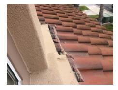
**5:-•** There is wood damage to the roof edge, under the eaves on the rear wood decking, indicating missing, broken tile, improper flashing or roof leaks at the edge. Recommendation: We recommend a licensed roofing contractor determine the reason for the damage, and repair the roof as necessary
