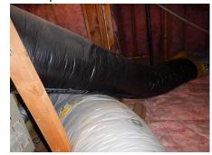
• The supply ducts are a modern, flexible type, comprised of a light-gray, plastic, outer sleeve and a clear inner liner that encapsulates fiberglass insulation, and those that were visible to us are in working order. However, the outer sleeve has been found to be susceptible to ultra-violet contamination, which causes the outer sleeve to deteriorate, and we recommend they should be monitored
