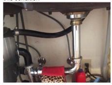
• The dishwasher is not securely mounted in the cabinet. This can lead to tipping, damage or injury. Recommendation: The unit be properly secured into the cabinet as required for safety
