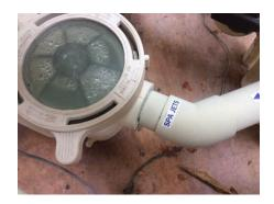
• There is a leak at the impeller housing of the spa boost pump motor. This indicates a loose or broken connection or housing. Recommendation: Service as necessary by a qualified pool specialist to restore leak-free operation
