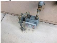
• There is no wrench at the gas shut-off valve to facilitate an emergency shut-off, and inasmuch as such tools are relatively inexpensive we recommend that you buy one and leave it in-place on the valve
