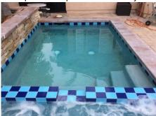
• The pool plaster is colored and mottled by calcium and other minerals leeching through to the surface, which is not uncommon with dark finishes. You may wish to discuss this condition with a pool contractor to determine if correction is warranted
