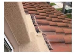
• There is wood damage to the roof edge, under the eaves on the rear wood decking, indicating missing, broken tile, improper flashing or roof leaks at the edge. Recommendation: We recommend a licensed roofing contractor determine the reason for the damage, and repair the roof as necessary
