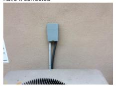
• The electrical conduit at the service disconnect is required to be attached to the wall within 12 inches of the box. This is to help prevent damage to the connection, and potential electrical hazards. We recommend the installation of proper wire restraint as necessary
