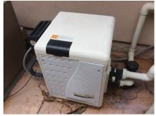
• There is water leaking from under the heater housing. This may be a drain plug or a more significant leak from the heat exchanger, as the water connections to this heater appear to be dry. Recommendation: The source of this water located and repairs made by a qualified pool contractor
