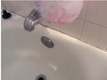
• The hand sprayer in the tub-shower leaks. this can lead to water intrusion and damage. Recommendation: Service as necessary to correct this condition
