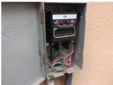
• The service disconnect is located directly above the coil. This is generally not recommended, as the disconnect should be accessible without reaching over the coil for safety. You may wish to have a specialist comment about this condition, or have it corrected
