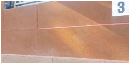
After Crack Repair & Caulk
