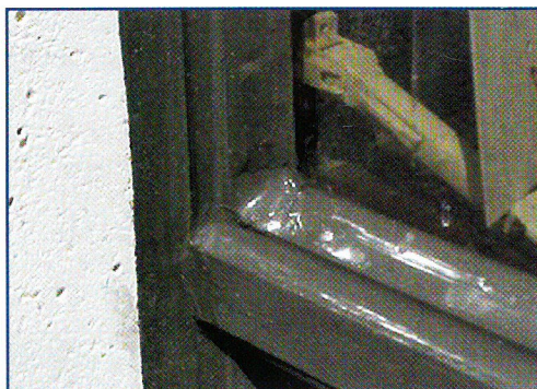
Figure 15 - Installed wet seal at window frame.
