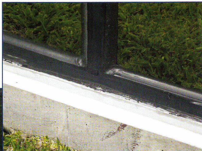
Figure 11 – Wet-sealed lockstrip.
