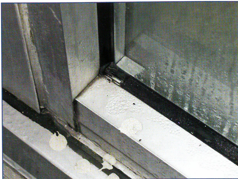
Figure 1 – Short gasket at corner of frame.
