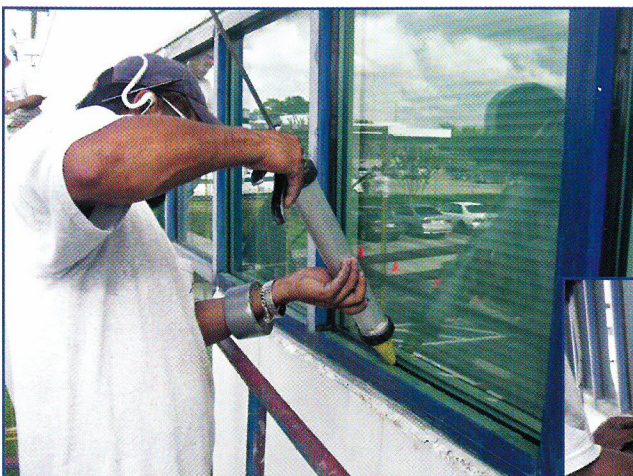
Figure 6 – Wet sealing window frame.
