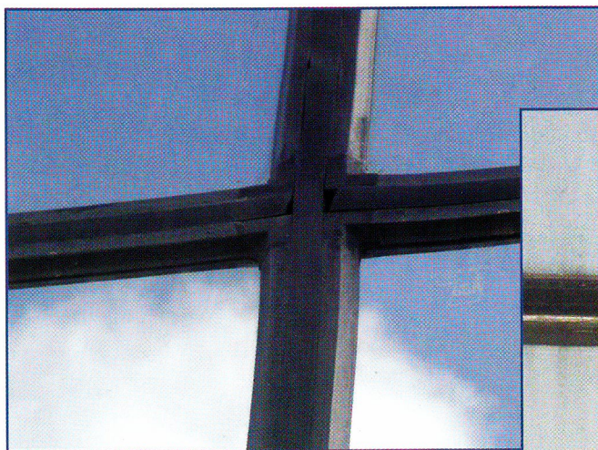
Figure 12 – Lock-strip gasket corner.
