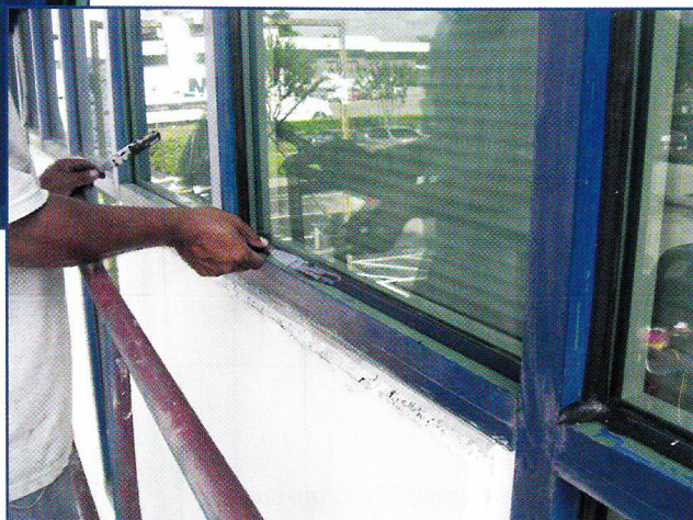
Figure 7 – Tooling sealant.
