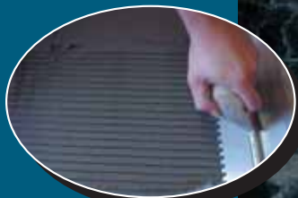
Apply Latex-Modified Thinset & Install Tile
