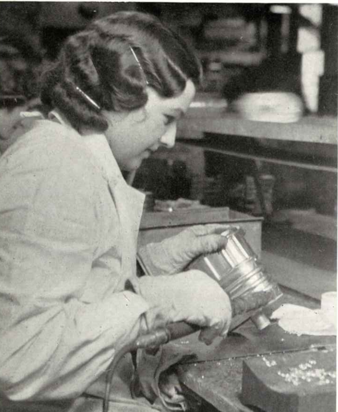
Soldering lid on to canister.
