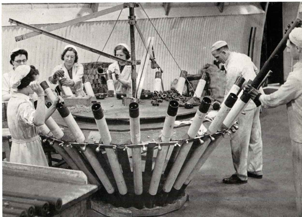
Filling Rockets with cordite on a "Roundabout."
