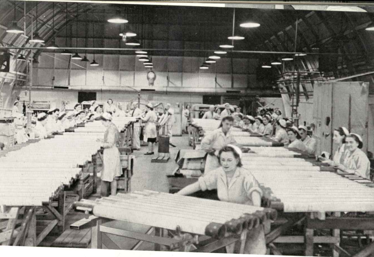
General View of the A.A. Rocket-Filling Shop.
