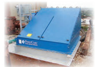
Torit PowerCore Model CPV-12 Cement silo bin vent conveyor (3700 cfm)
