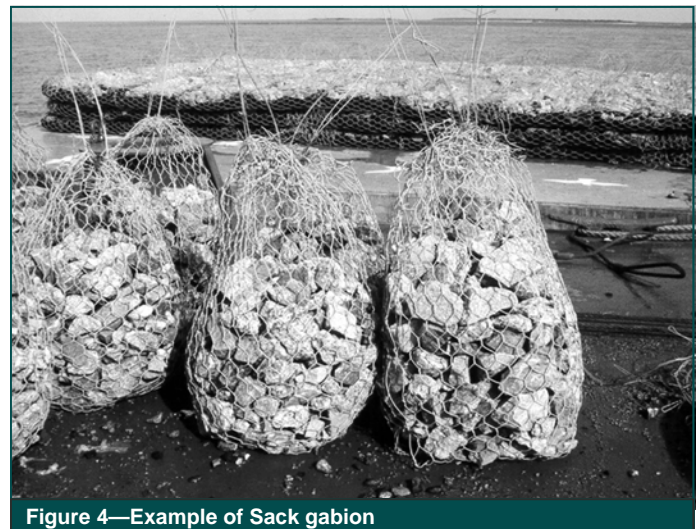
Figure 4—Example of Sack gabion
