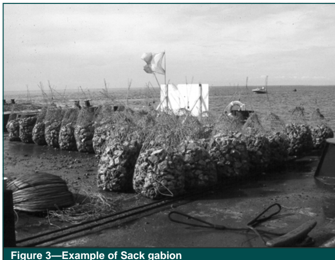
Figure 3—Example of Sack gabion
