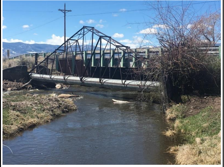
Diversion dam on feeder ditch
