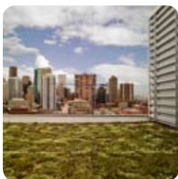
Green roof atop the EPA Region 8 office in Denver, CO. Photo courtesy of Greg Davis.
