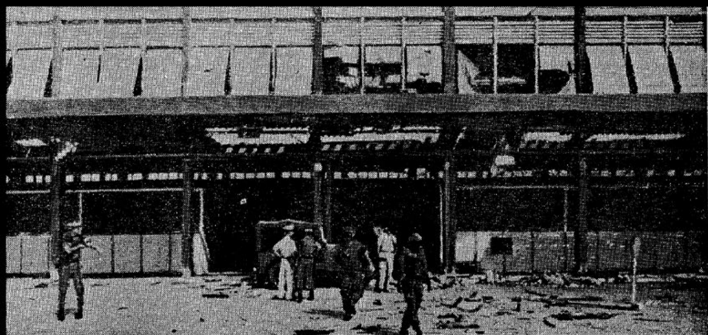
Vietnamese authorities look over rubble scattered on the ground outside the Tan Son Nhut Airport terminal after the building was shattered by a Viet Cong bomb. At least 46 persons, including 36 U.S. servicemen, were injured. (AP Radiophoto)
