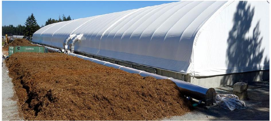
**Aerated static pile composting takes place in a fabric building. Exhaust air is pulled through the adjacent biofilter.**
