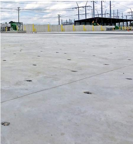
**Newly built sparger type floor for the positive aeration mass bed used for curing (foreground). Active composting bunkers and preprocessing building (on far right) are in the background.**
