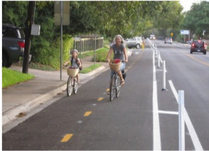
Separate two-way bike lane with bollard indicators.
