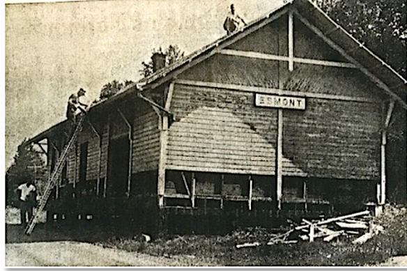
Esmont Depot Being Dismantled, 1964
