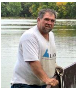
Juice Langowski at the dam preparing to weld the carp barrier together.
