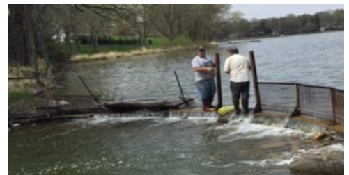
Juice & Doug position key pieces of the new carp barrier prior to welding. →
