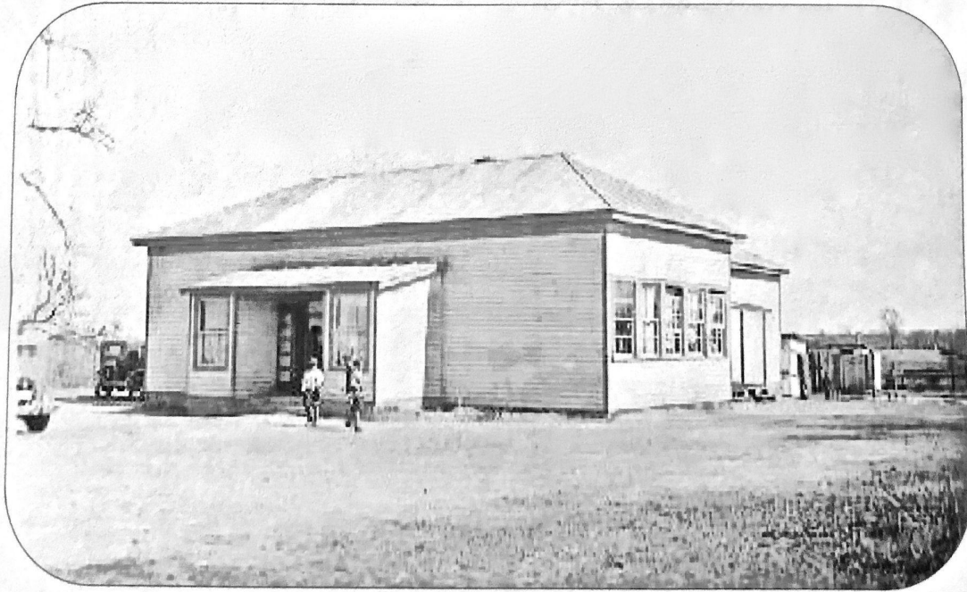
Built in 1925 with additions in 1928 and 1930, four classrooms
